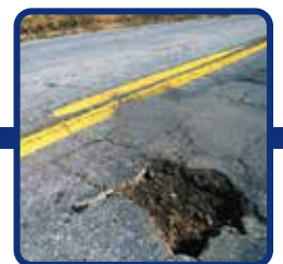
POTHOLE/DAMAGED PAVEMENT
